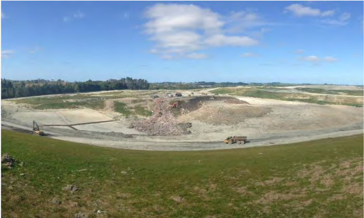
Figure 2: Redvale Landfill – Wholly owned and operated by WMNZ Ltd.
